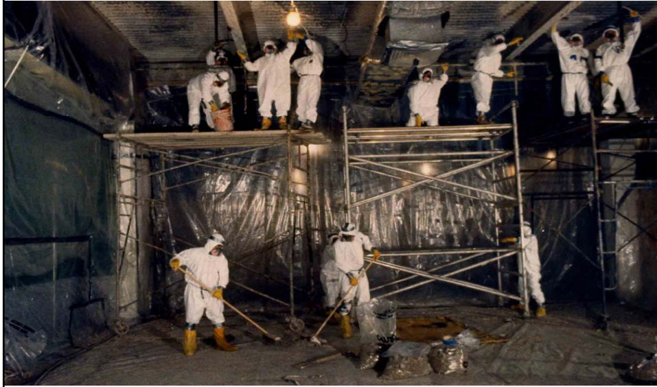
Fire Proofing Abatement Project
